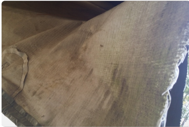
Mold forming on the inside of a cover due to lack of air-permeability.
